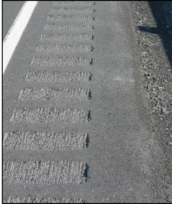
Figure 24: Shoulder Rumble Strips 31
