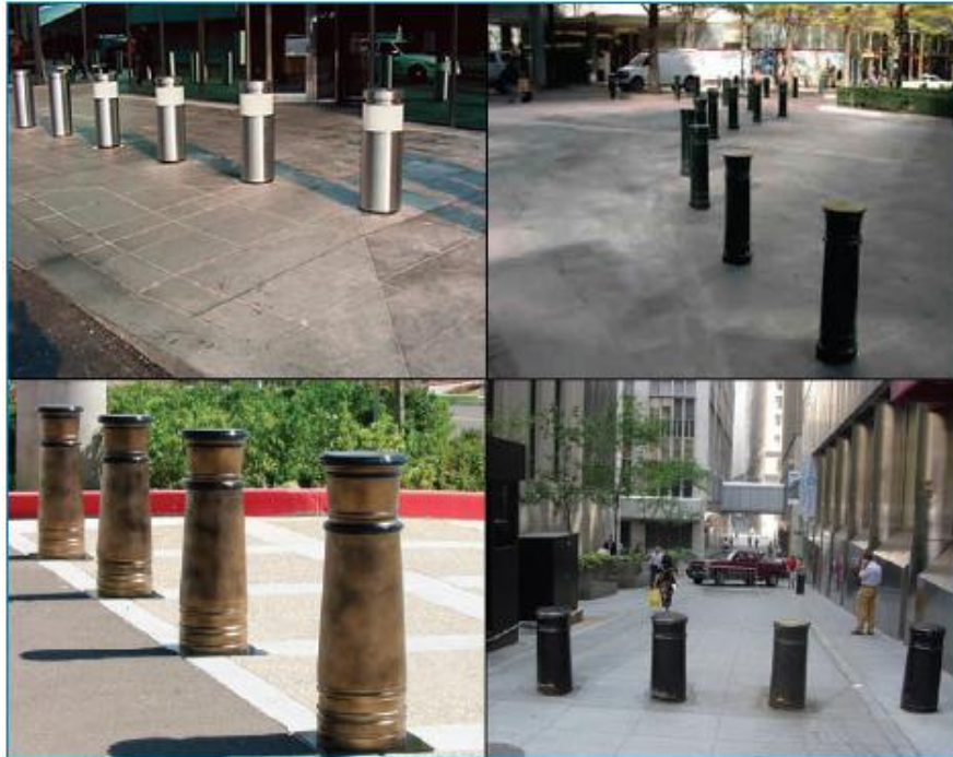
Figure 2: Decorative bollards with high-performance ratings.
