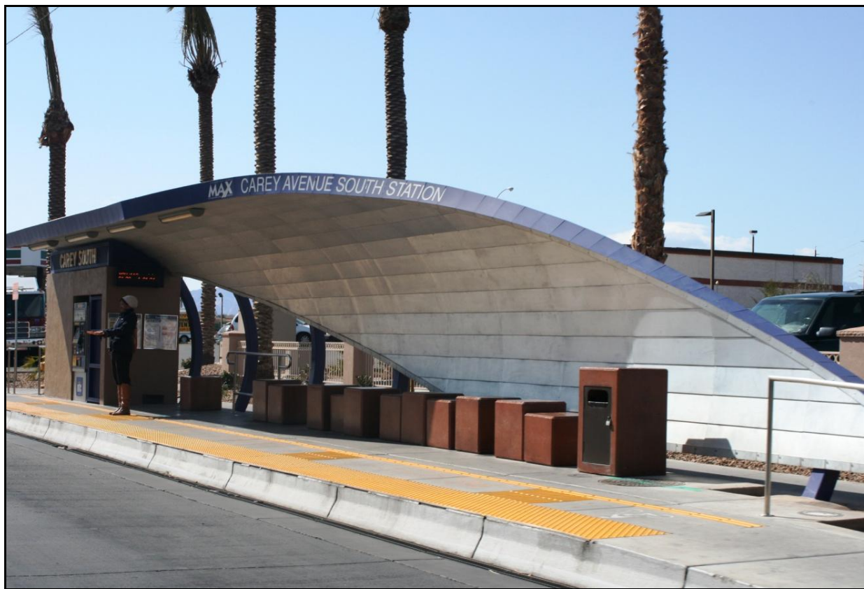
Figure 10: Raised Curb At Las Vegas MAX Stop
