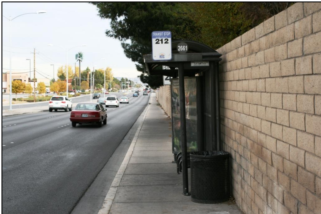
Figure 7: Las Vegas Valley Transit Shelter Located Against A Block Wall
