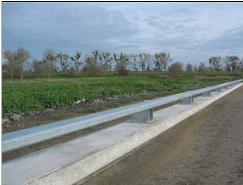
Figure 14: Caltrans' "Test" Low Profile Barrier 19
