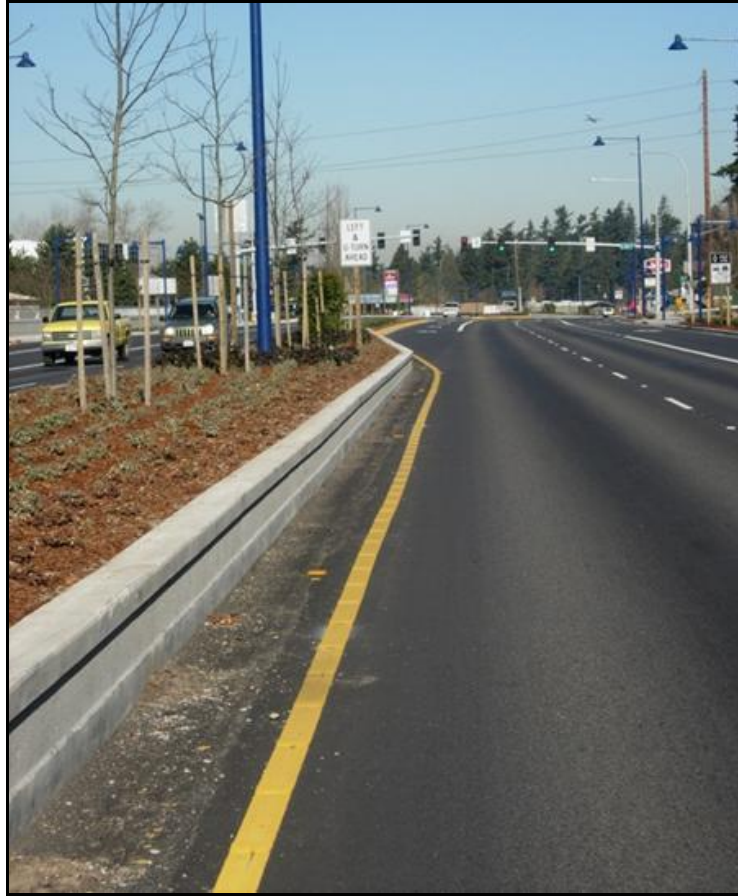
Figure 13: Low Profile Barrier In Des Moines 18
