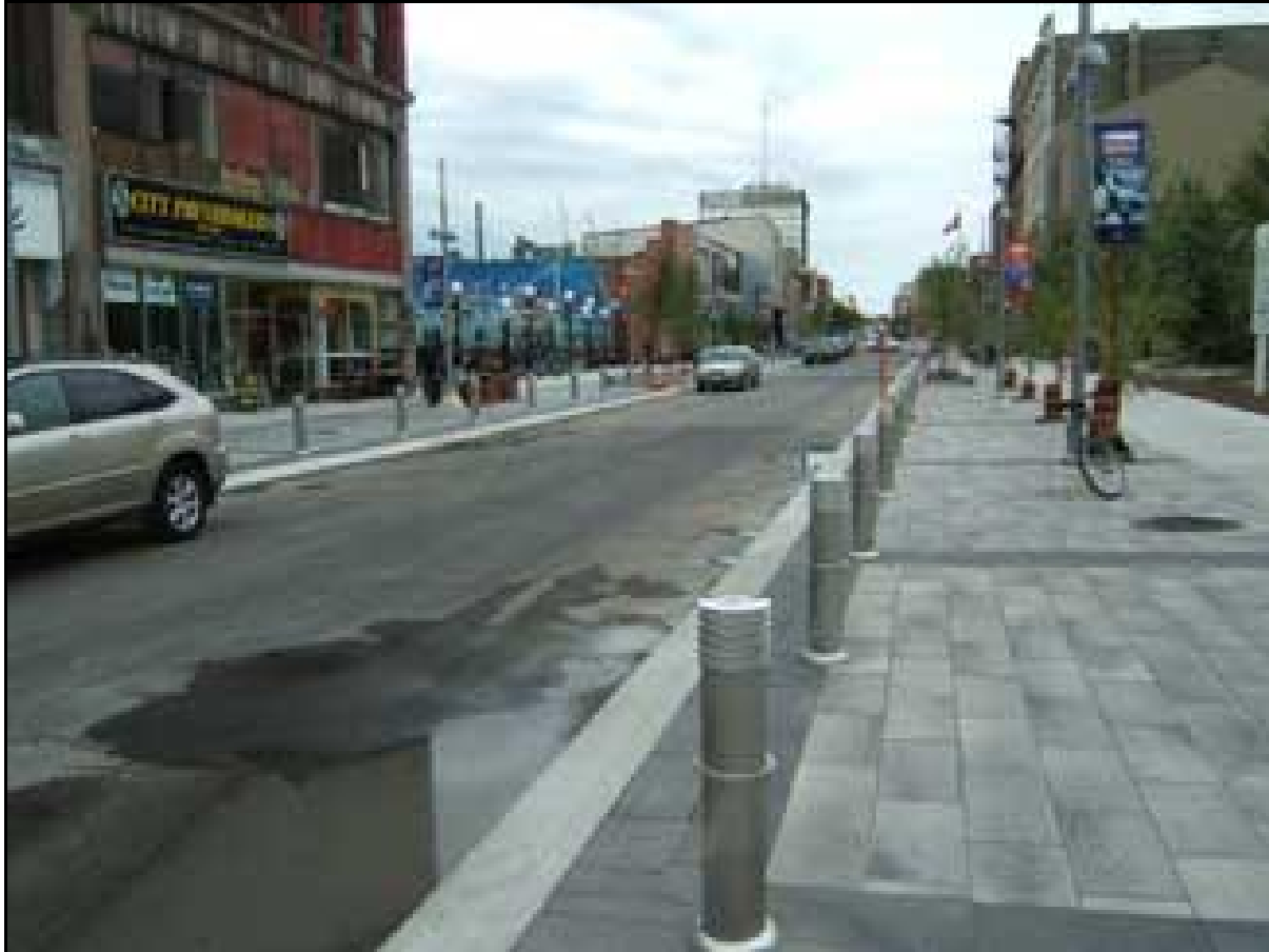
Figure 15: Bollards Separating The Roadway And The Sidewalk 23
