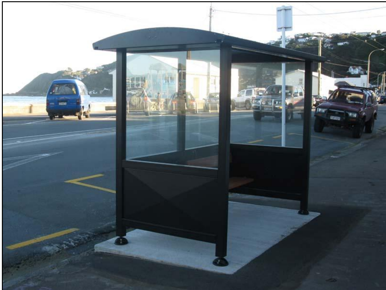
Figure 28: Rear-Facing Transit Shelter 35
